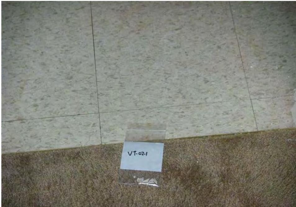
**Sample No. VT-02-1, Asbestos-Containing Vinyl Floor Tile (tan 12"x12" with brown/white streaks) with Mastic (black).**
