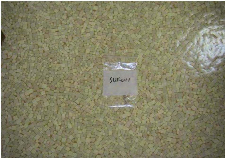
**Sample No. SVF-04-1 and SVF-04-2, Asbestos-Containing Sheet Vinyl Flooring (tan/grey with brown grout square terrazzo pattern) with Non Asbestos-Containing Mastic (yellow).**
