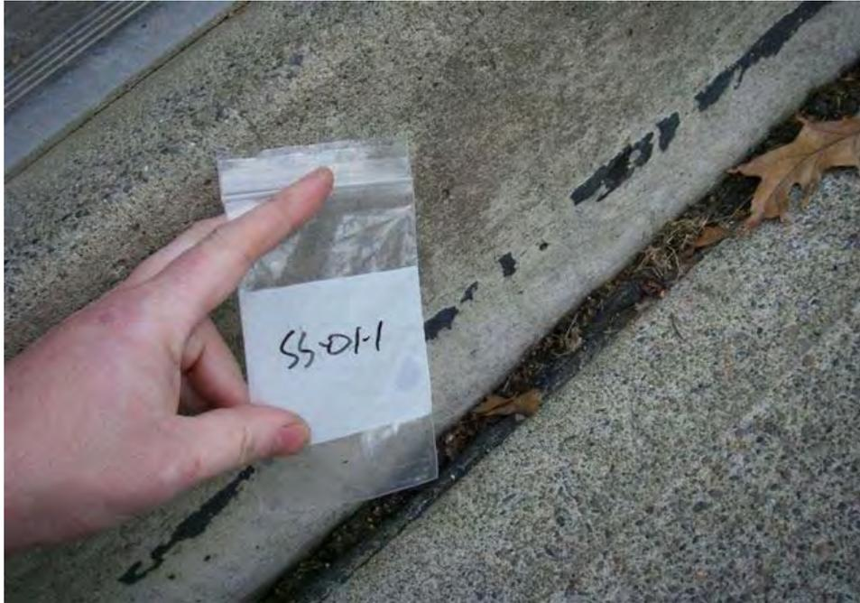
**Sample No. SS-01-1, Seam Sealant (black on concrete joints).**
